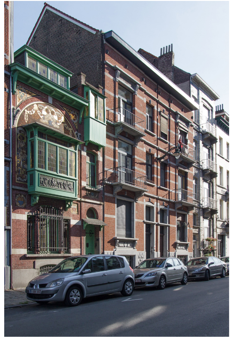
Brick town houses
