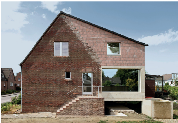
fig. 2 Façade of Haus Schreber by AMUNT architecten (Dujardin, n.d.)
