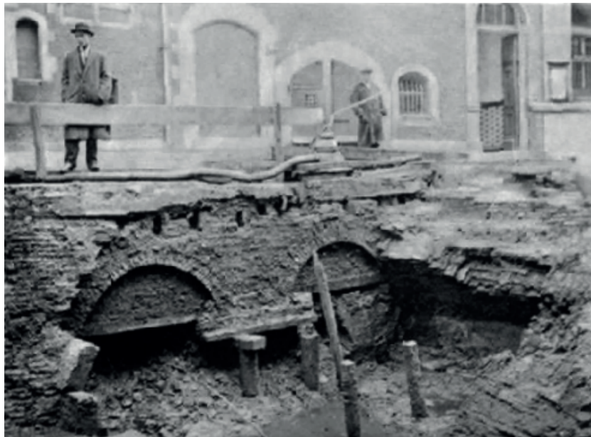
Figure 3.3: Masonry pipe named the "Oude Spoye" being excavated, which mouthed in the "Rokin" channel (Bakker, n.d.).
