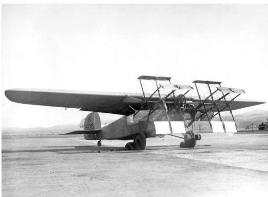
Figure 3.30: Schroeder S1 Cyclogyro (1930), from Schwaiger [75]
