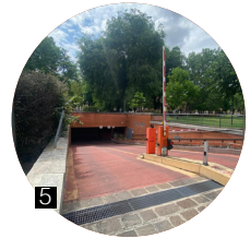
Underground parking lot
