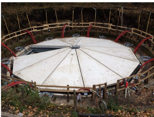
Fig. 3. Construction of the real Ecovat system.
