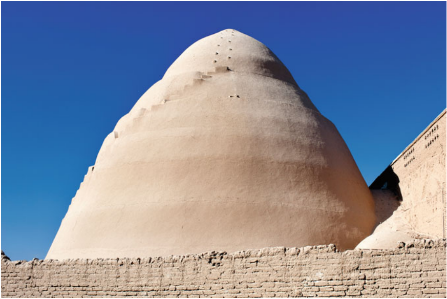
An ice house, yakhchal , like this one in Meybod, was used to store ice in underground chambers throughout the year, Wikimedia, Ggia, released under a Creative Commons Share-Alike 3.0 license
