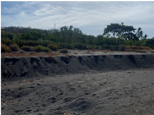
Figure 3.22: Beach scarp at transect 44
