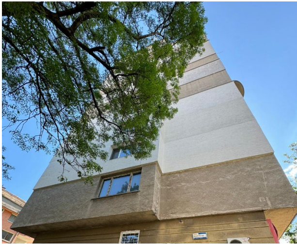
Figure 13: Partial Insulation Improvements in a Communist Flat (Photograph: taken by author)
