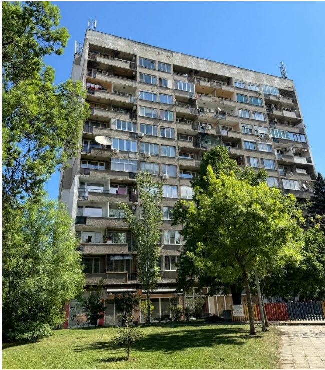
Figure 9: Image of a Residential Flat with a Park next to it (Photograph: taken by author)
