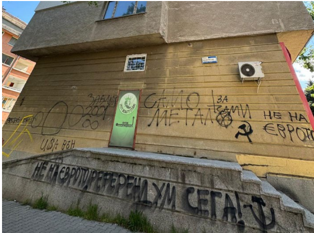
Figure 12: Graffiti on Old Communist Buildings (Photograph: taken by author)
