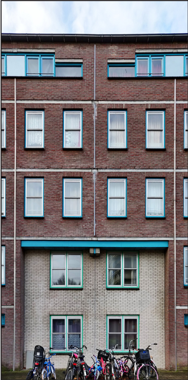
Figure 4. straight-on picture of the north-east facade
