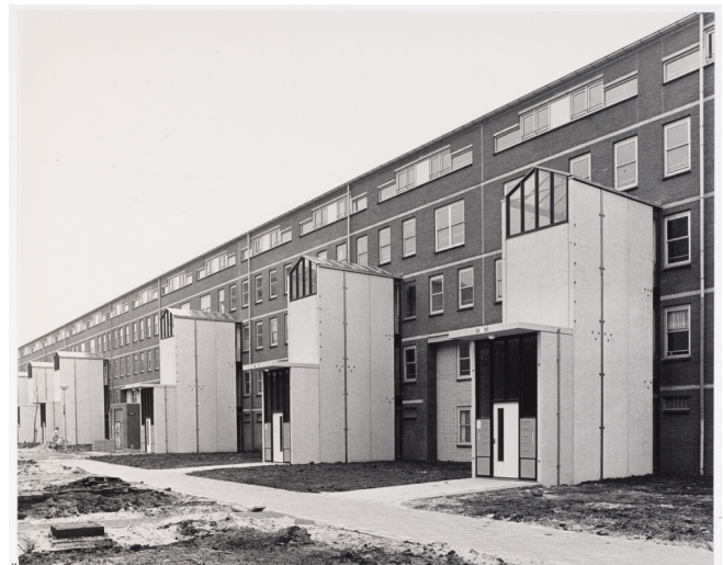
Figure 2. East side of the building with new staircases in front of the original back side of the building. From “Stadsarchief Amsterdam”, by Archief van de Gemeentelijke Dienst Volkshuisvesting, n.d.
