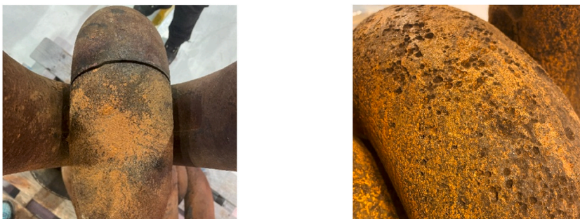
Fig. 1. Fatigue crack (left) and corrosion pits (right) in mooring chain links.
