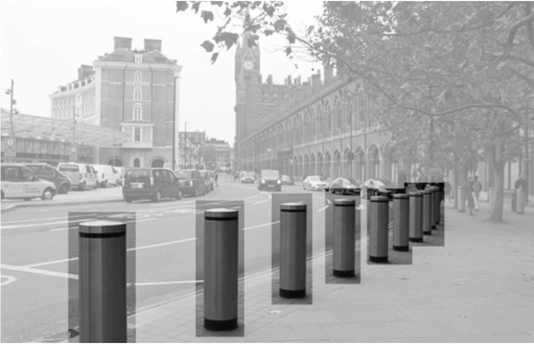
King's Cross Station, in front of Pancras Square
