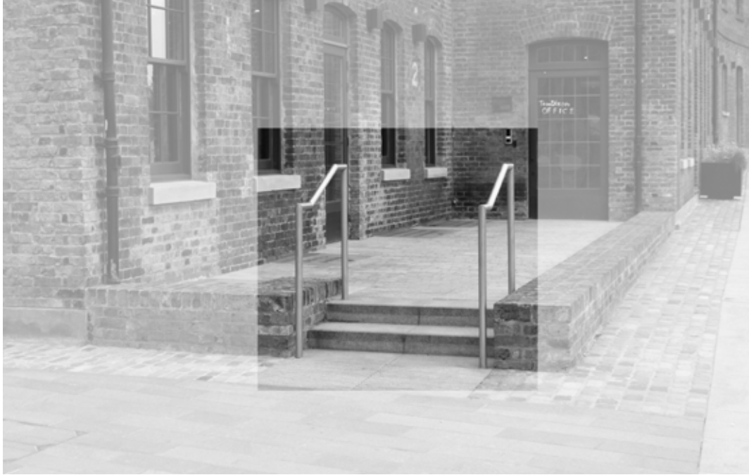
Granary Square Concrete staircase with steel handrailing Transition and safety element
