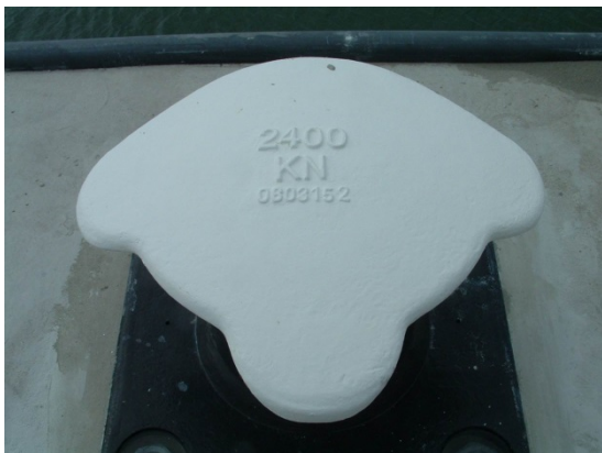
Figure 6. Standard 2400 kN bollard Rotterdam
