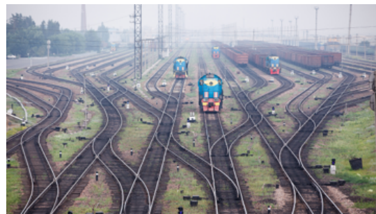
Figure 1.6: A view on the complexity of railway infrastructure [20]
