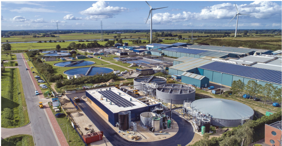
Figure 11.17 The Nereda ® plant in Zutphen, the Netherlands with a Kaumera-extraction plant. In the background is the existing conventional activated sludge plant.
