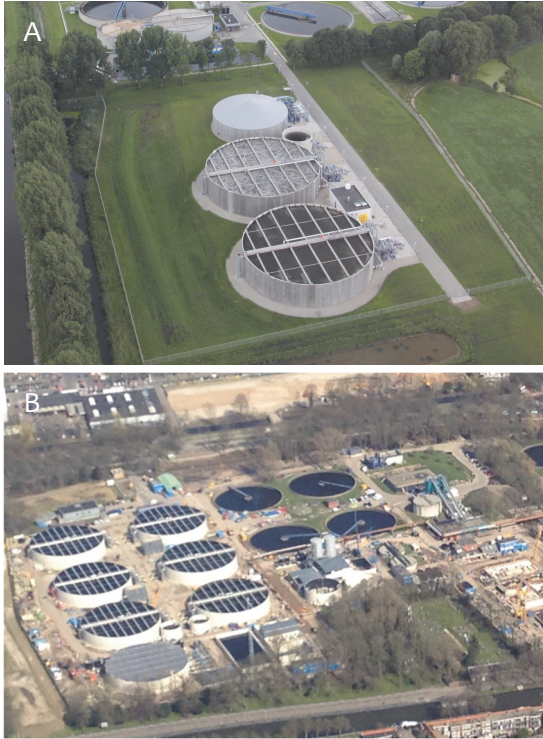
Figure 11.1 Nereda® wastewater treatment plants in the Netherlands in (A) Garmerwolde (140,000 P.E.) and (B) Utrecht (430,000 P.E.). In Utrecht the new 6-tank Nereda® facility (in operation since 2019) is visible on the left with part of the old abandoned plant on the right.
