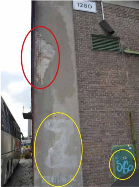
Figure 32 - Damages East facade - Own Illustration
