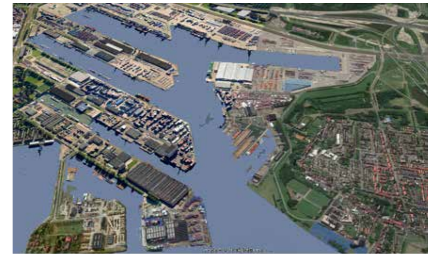
Aerial view of Eemshaven
