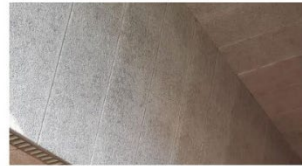
fiberboard ceiling panels in the courtroom
