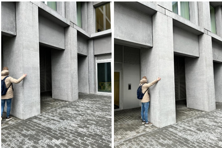
columns at residential tower new south by DRDH
