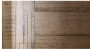
concrete bearing walls with pattern of the wooden formwork
