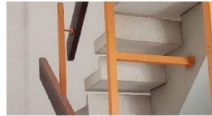
orange colored balustrade with simple wooden handrails
