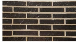
glazed interior brickwork in the main hallway
