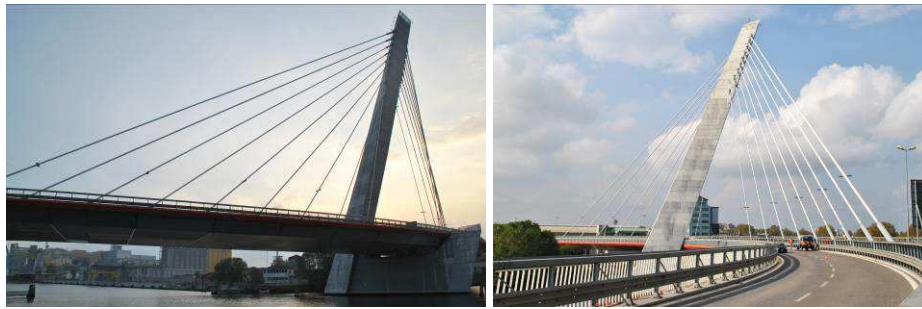
Fig. 1 Views of the curved cable-stayed bridge in Porto Marghera (Venice, Italy).
