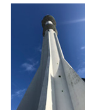
Transmission tower Rotterdam Harbour Author, 2020
