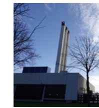
Cooling Facilities Data Center Rotterdam Author, 2020
