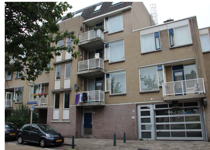
Van Leeuwenhoekstraat是Vestia协会在海牙的一个社会住房项目，该项目每套住房面积约55平方米，距离海牙市中心1.5公里。 Van Leeuwenhoekstraat is a social housing project of the Vestia Institute, which is 1.5 km away from the center of the Hague, with 55 square meters of each house.
