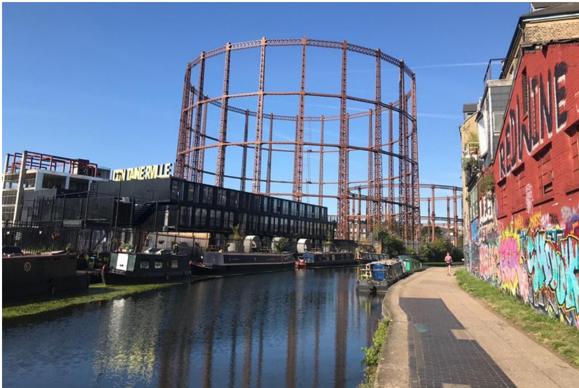
Photography 2.3: The "Oval Space": View at the gasholder from Regent's Canal
