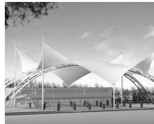
Arch-type membrane
