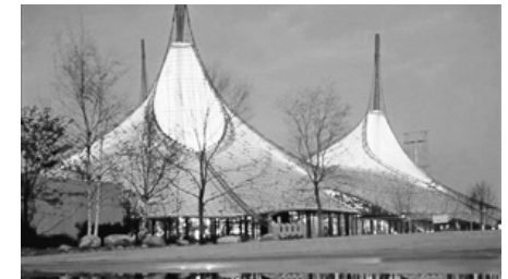
High-point-type membrane
