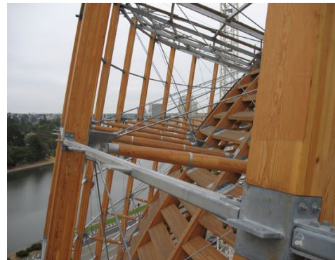
Cable in tension
