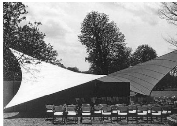
Simple saddle membrane
