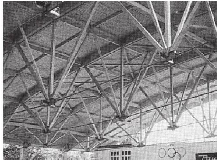
Fish belly truss with steel tie
