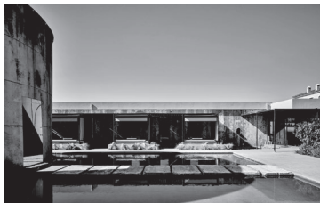
Concrete blocks divided for wine storage tanks (5m x 6m) used as hotel rooms. Doorway openings - slabs used as stepping pathway.
