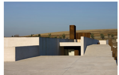
Use of white concrete and rusted steel i.e. contemporary materials that communicate with stucco and ceramic of the ancient city.
