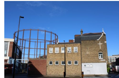
View from Hackney Road The lightweight structure of Gasholder No.5 seen in the background gives a glimpse of the industrial heritage of the area while contrasting with heavy brick building in the foreground.
