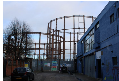
View from Marian Place Gasholder No. 2 and 5 seen from the previously used main entrance of the gas storage station site
