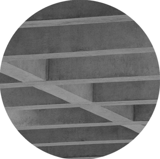
ribbed concrete slabs
