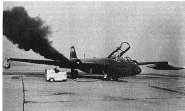
*Figure 3: B-57 modified to use liquid hydrogen (Sloop, 1977). The heavy smoke was a normal occurrence during engine startup on conventional fuel.*
