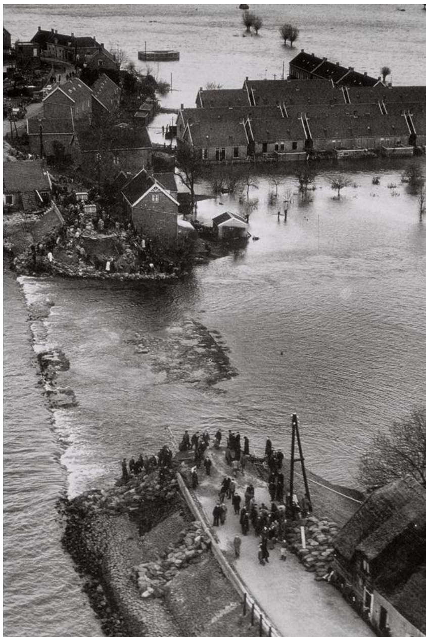
Figure C.2: Levee breach at Den Bommel in South Holland, as a result of the 1953 storm. Image source: https://beeldbank.rws.nl , Rijkswaterstaat
