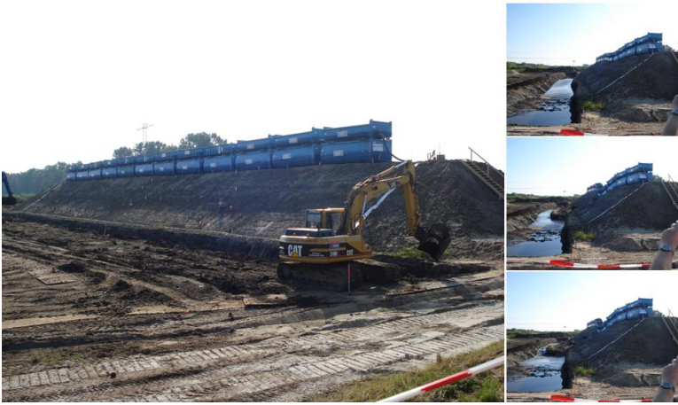
Figure 6.14: The macrostability field test on the IJkdijk in 2008.
