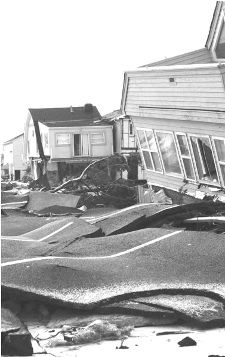
Figure 6. Long Beach residences damaged after Hurricane Sandy, 2012.
