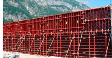
Figure 2-6 - System formwork (directindustry.es)
