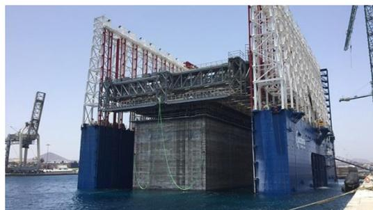
Figure 2-21 - Use of a floating dock to construct a caisson (acciona-construccion.com, 2018)
