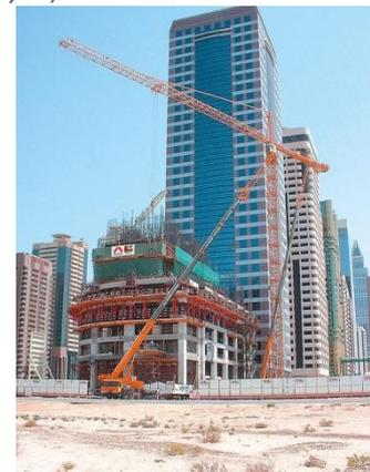
Figure 2-7 - Crane-climbing formwork (peri-usa.com)
