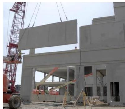
Figure 2-4 - Prefab concrete structure
