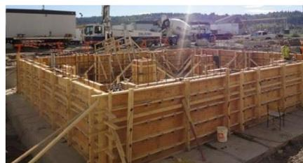
Figure 2-5 - Traditional formwork
