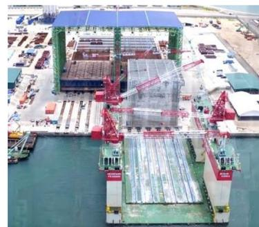
Figure 2-19 - Transportation of caisson on semi-submersible vessel (Krabbendam, 2016)
