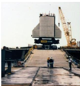
Figure 2-1 - Use of caisson as bridge pier ([severnbridges.org](http://severnbridges.org))
