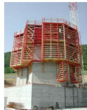
Figure 2-8 - Self-climbing formwork at bridge of Millau (engineersireland.ie)
