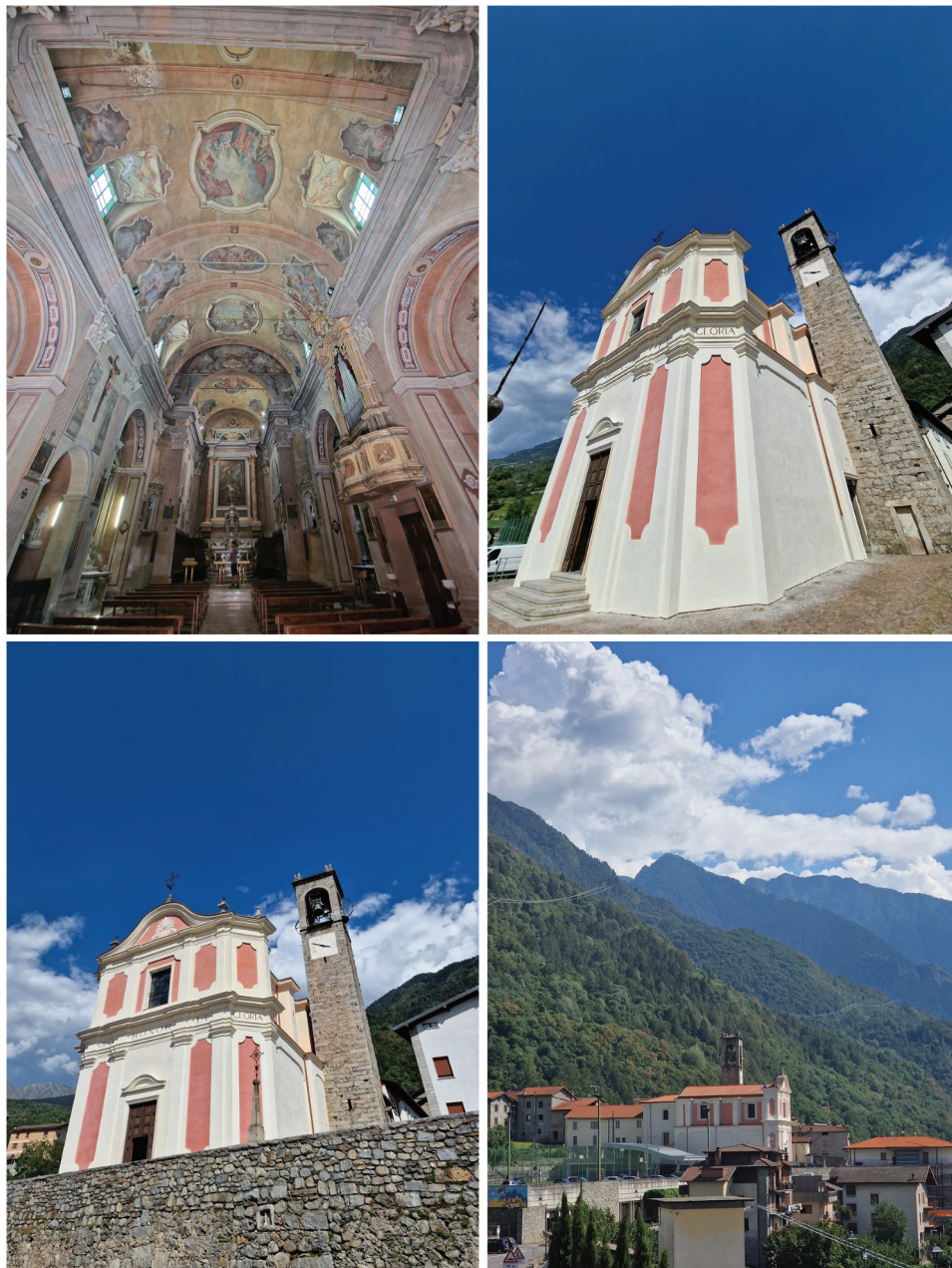
Figure 9. Views of the church of Ceto after the seismic retrofitting and restoration work.
