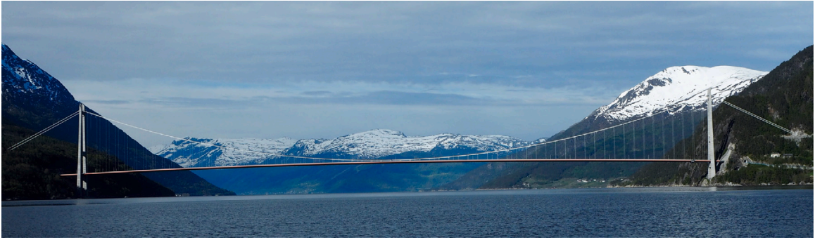
Fig. 3. The Hardanger Bridge (Photo: Aksel Fenerci/NTNU).
