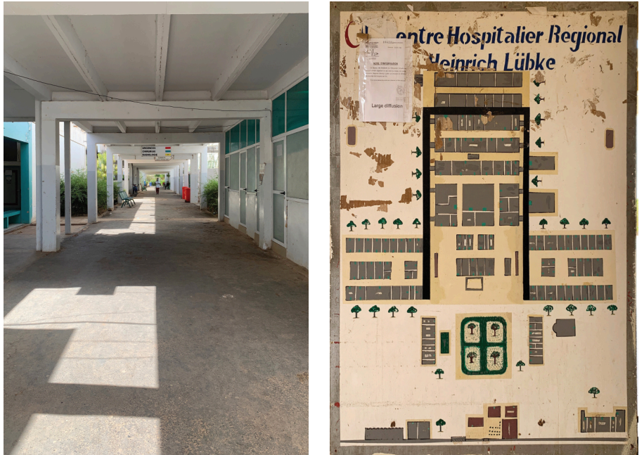
Figure 3b-c: Heinrich Lübke Regional Hospital in Diourbel, Senegal, architect: Lippsmeier + Partner. State: May 2022.
