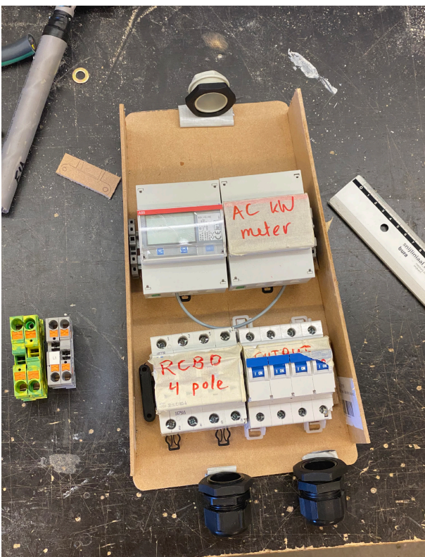
Figure 62. Component configuration that would not fit. ▼
