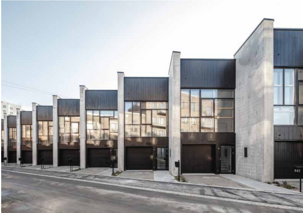
Upcycle Studios, Øerestad, Copenhagen, 2018 (by Lendager) built from recycled concrete, repurposed double glazing windows and discarded flooring boards. https://lendager.com/project/upcycle-studios/
