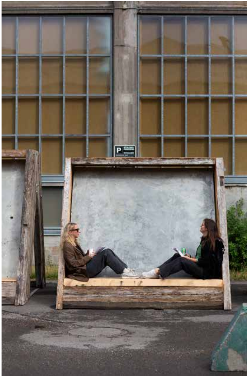
(P)RECAST UIA Pavilion, Copenhagen, Denmark. Modules of sourced concrete walls framed by demolished 200-year-old timber beams (by GXN). ( https://gxn.3xn.com/project/pre-cast-uia-pavilion )
