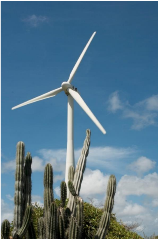
image (32). Wind turbines. Photo from eventscuracao.com/the-wind-turbines-of-curacao/
