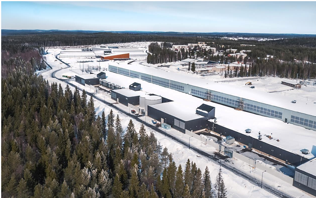
image (12). Data centre in Luleå, Sweden. Photo by Meta
