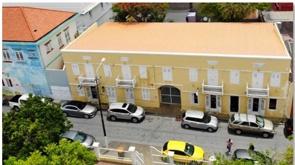
image (69). In contrast to the extrovert courtyard (image 68), the architectural design is introverted on the street side. Photo from stadsherstel.com/van-raderstraat-9-23-2/
