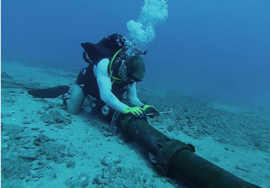
image (11). Repairing submarine fibre-optic cables. Photo by U.S. Pacific Fleet
