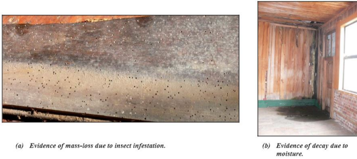
Figure 3.13: Deteriorated condition of vintage Whanganui timber diaphragm tested in-situ.[32]
