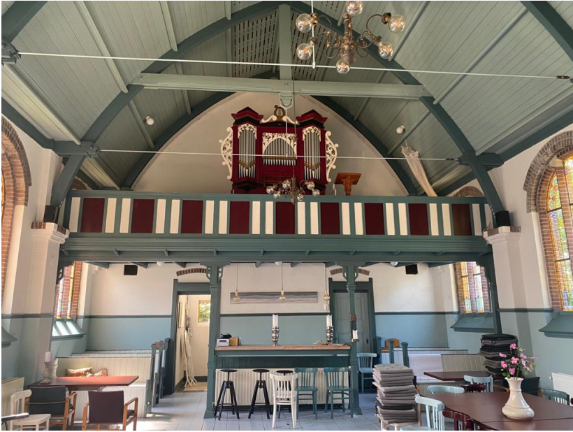
Figure 5.6: Installation of 4 new columns supporting the first floor in the main-structure (site visit,2021)
