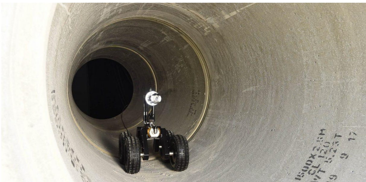
Figure 1. CCTV Pipe inspection (Allpipe, 2020).
