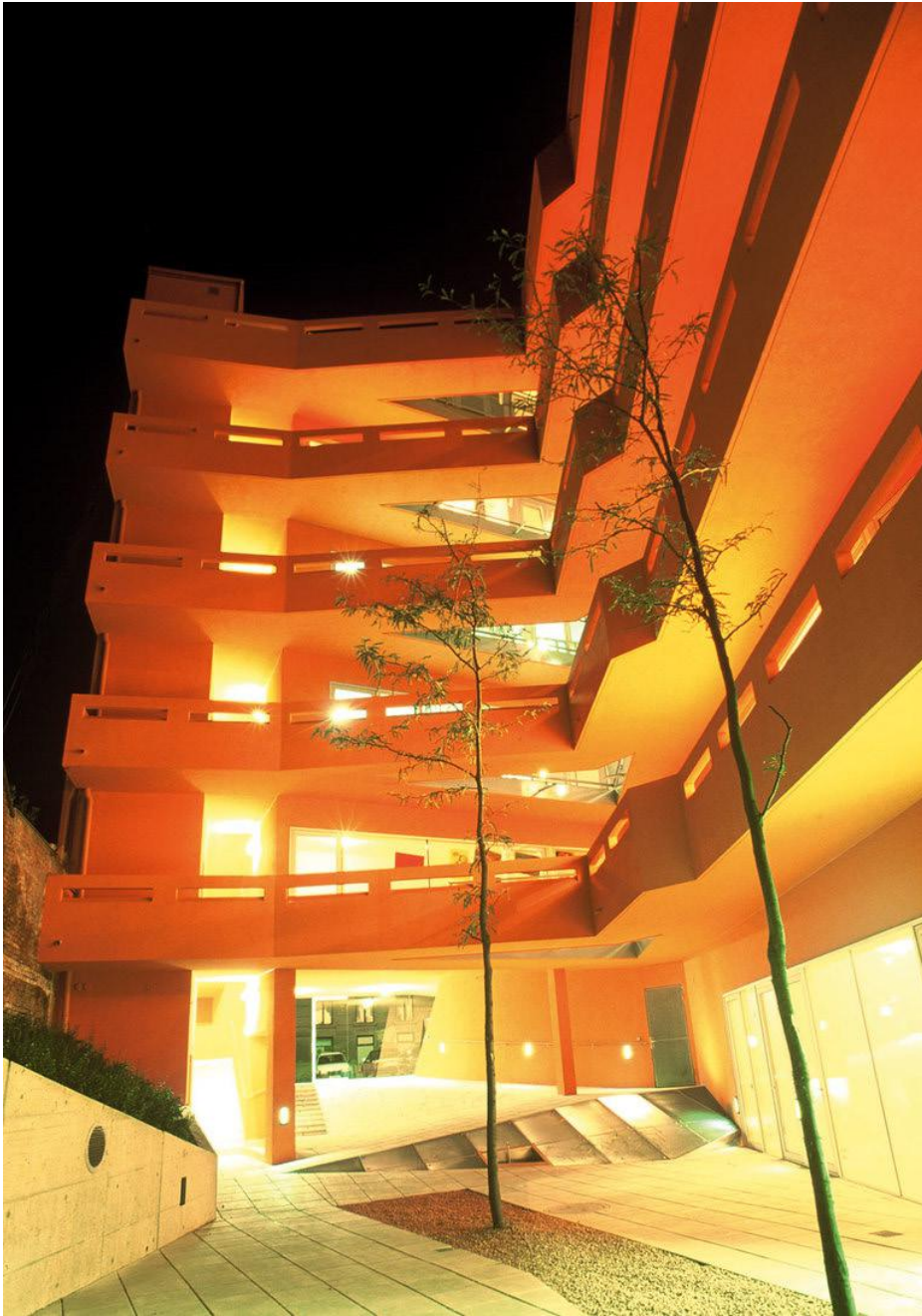
Fig1.3.1: Miss Sargfabrik , Gallery seen from courtyard Photo © Herta Hurnaus
