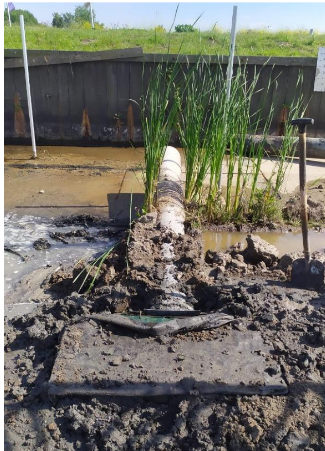
Figure 82: Excavated tube with infiltration box
