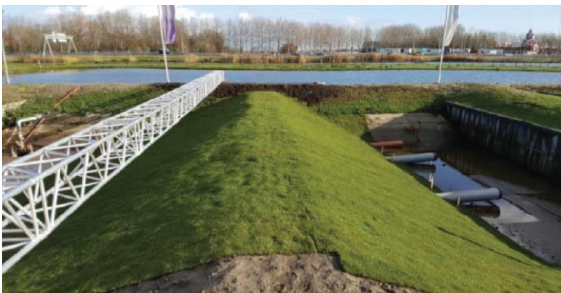
Figure 84: FPH dike right after construction (Picture by Joost Pol)
