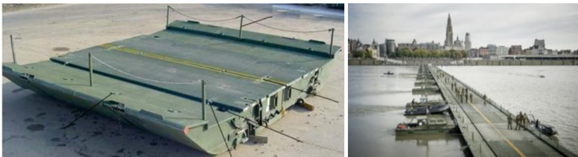
Figure 2: Pontoon used as temporary bridge element
