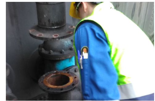
Executed lockout out for pipe replacement
