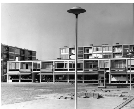
*1965-69 two-storey residential-commercial housing block
