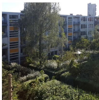
3. Two years later in September 2016 the bushes were grown but the residents did not put much effort to maintain the garden.
