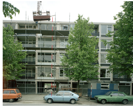
*Figure 1.3.16. 1984: Being renovated with plastic window frames
