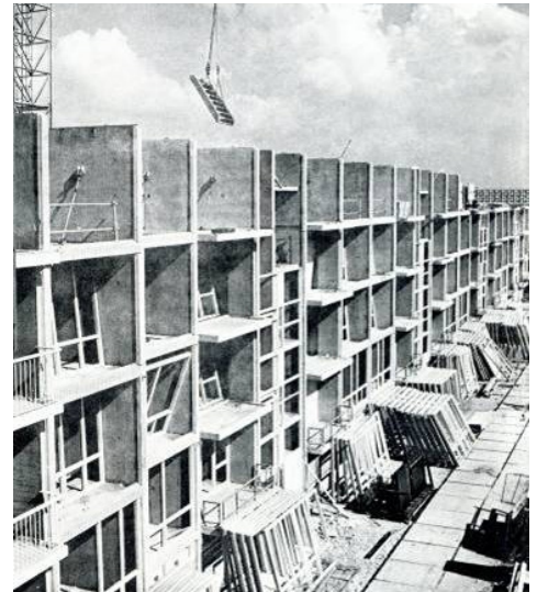
Figure 1.2.3: Assembly on site
