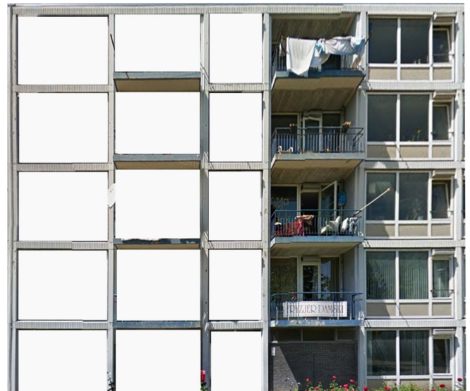
Figure 1.3.4. Comparison between a skin with the grid only and with both grid and infill
