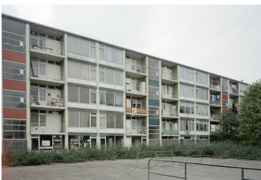
*1984 wooden window frames of the facade (before the renovation)
