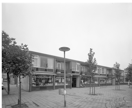
*1983 two-storey residential-commercial housing block
