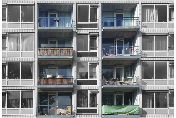
Figure 1.5.50 appearance from outside
