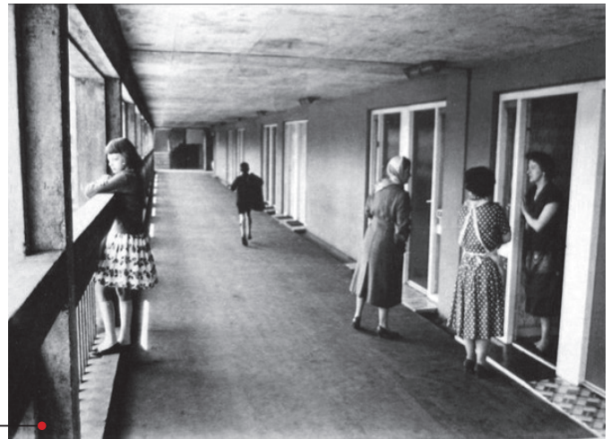
Figure 2.2.10. Original walkway: a communication space (Municipal Dreams in Housing, Sheffield, 2015)
