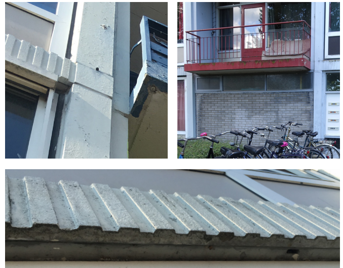
Figure 1.3.5 . Prefabricated fragments attached to structure
