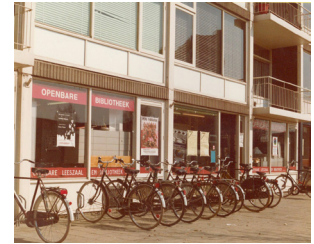
*Figure 1.3.20. 1973-78: Vertical grid painted white; Horizontal grid painted brown; Window frames and parapet white.
