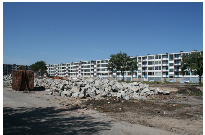
Figure 1.1.17 Demolition of the Intervam flat in Donaudreef. (Photo link: http://mapio.net/s/42073773/ )
