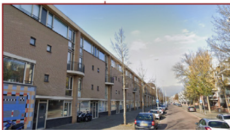
New Low Income Flats - Built 2000's, Mid size and cheap
