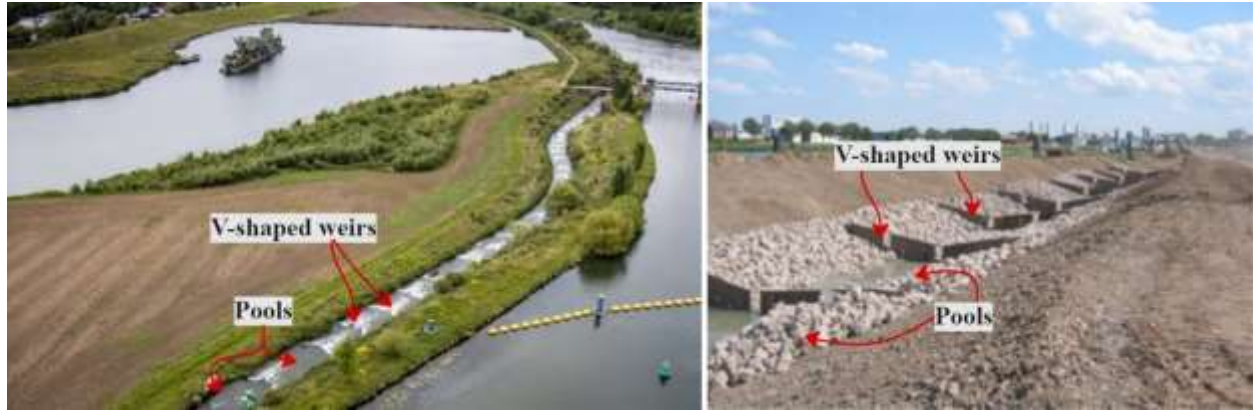
Figure 5: V-shaped pool-and-weir fish ladder at weir complex Borgharen (Rijkswaterstaat, n.d.) and (Vriese, et al., 2021)
