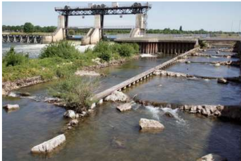
Figure 65: Overview of the fish ladder at Sambeek (Buiter, 2020)
