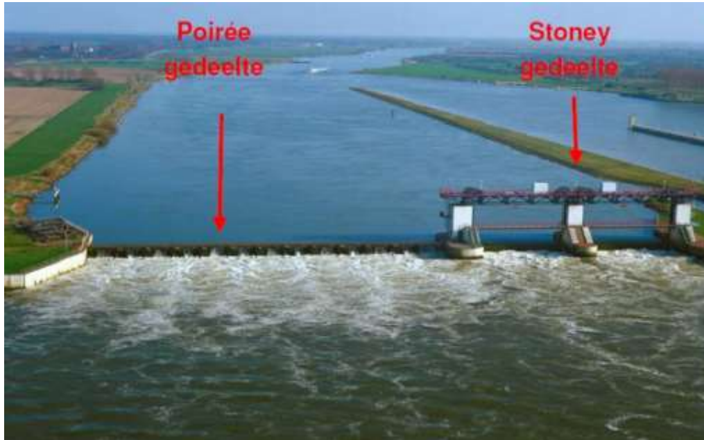
Figure 63: Overview of the combined Poirée and Stoney weir at complex Sambeek (Heer, 2020)
