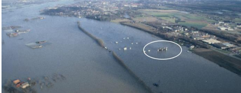
Figure 11 Weir structure during high flow, source: Rijkswaterstaat
