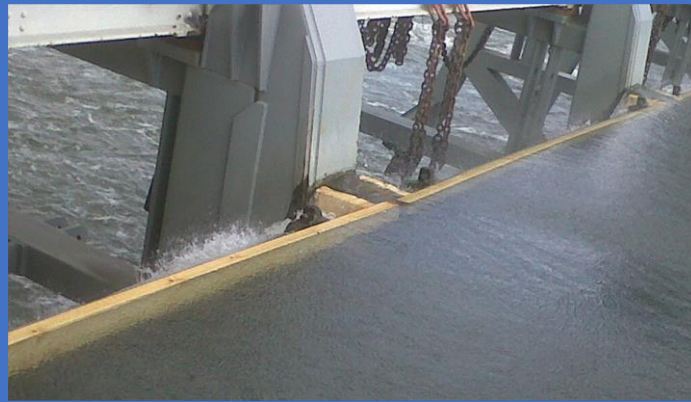
Figure 12 Improvised beam on top of weir Sambeek, source Rijkswaterstaat Henry Veugelers
