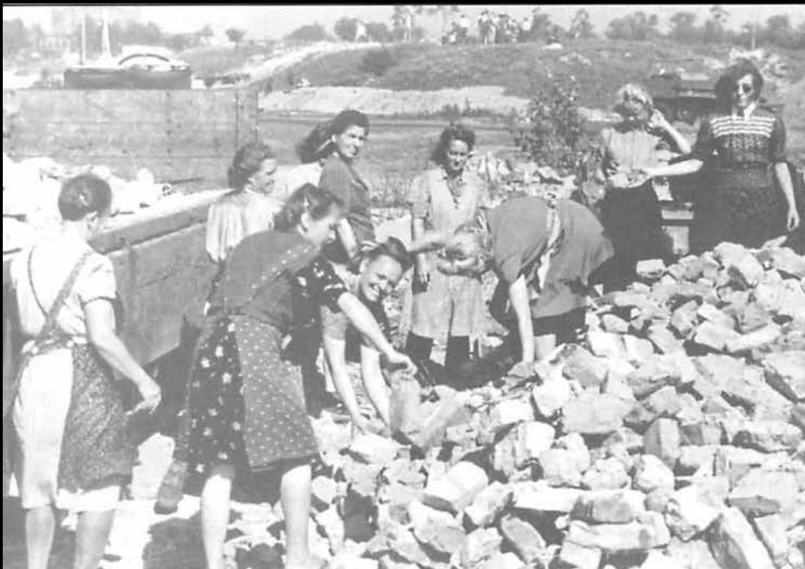
TXL CONSTRUCTION SITE, 1948
