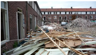
Fig. 13: Start of Demolition at the Copernicuslaan
