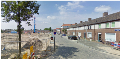
Fig. 11: Copernicuslaan, during demolition
