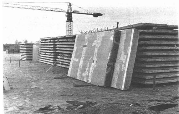
Figure 19: Stock piling at the construction site, source (Dijk et al., 2000)
