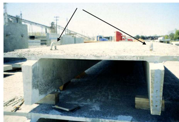
Figure 16: Lifting eyes of a prefabricated double-T beam, source (Levitt, 1990)
