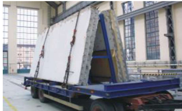
Figure 20: demolition site to storage facility, source: (Glias, 2013)
