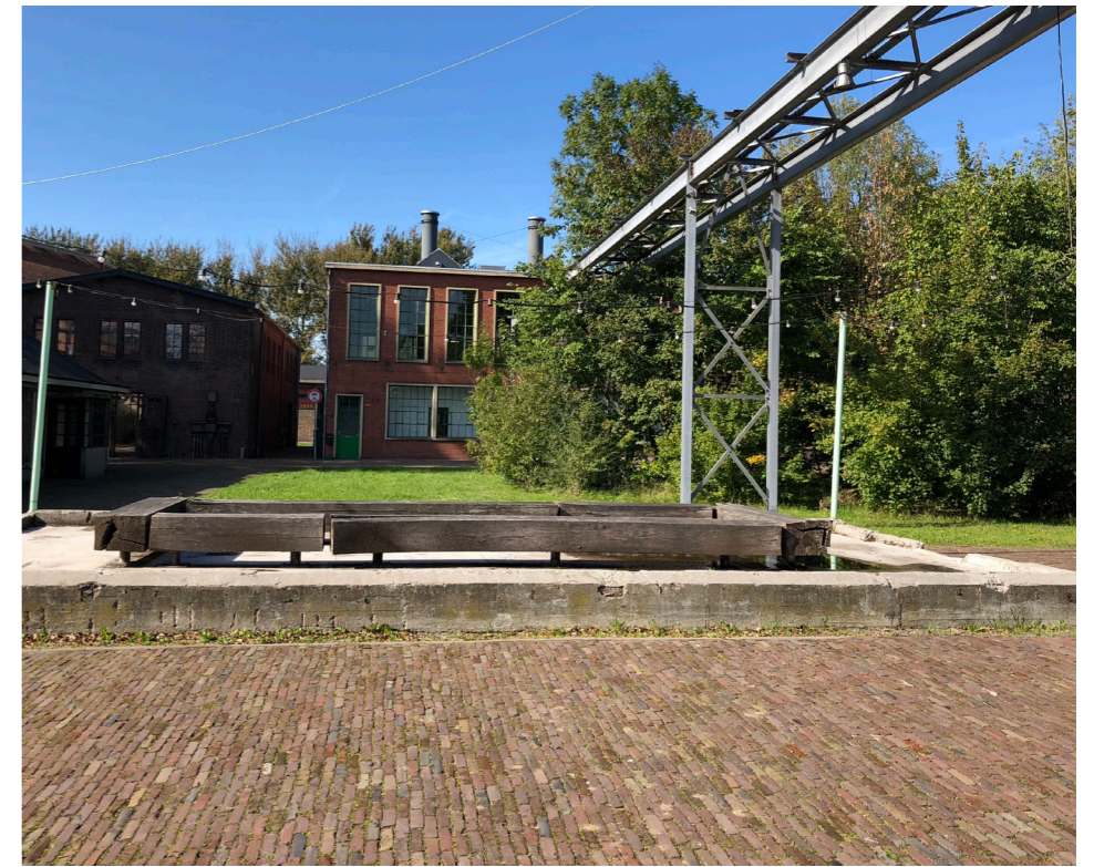
Steam pipe axis
