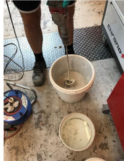
b) Mixing of gypsum
