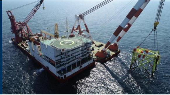
Fig. 3 Vessels during Jacket installation
