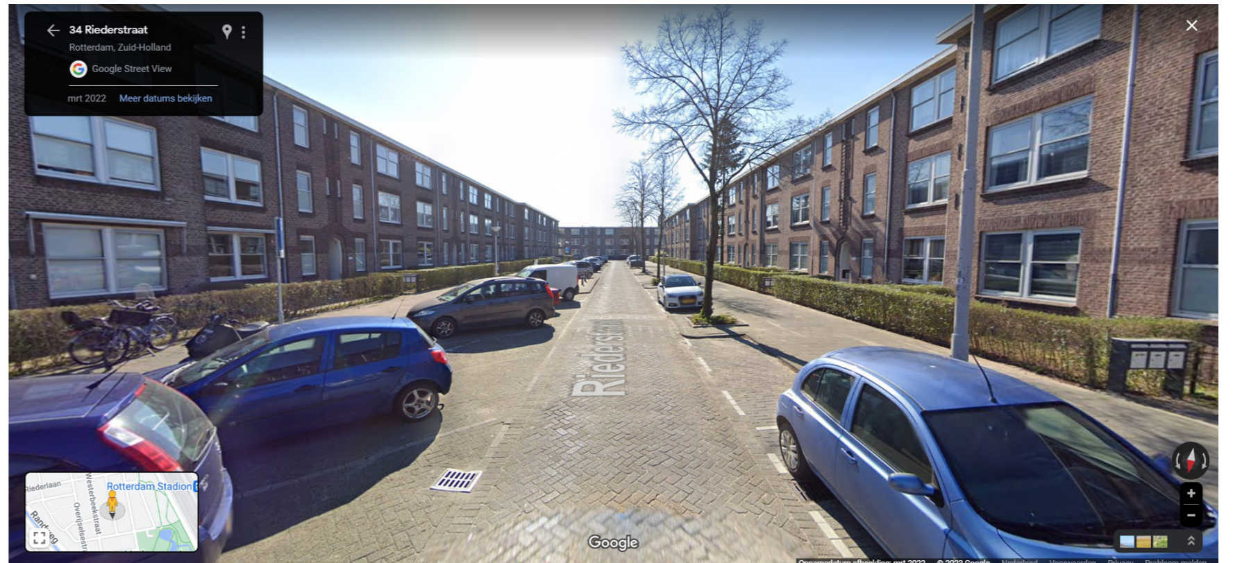
5.26 - Hillesluis street, before
